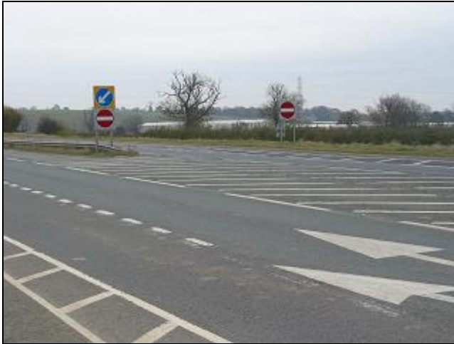
Figure 4: Road signs, industrial units and pylons at the western end of the Malton bypass.
